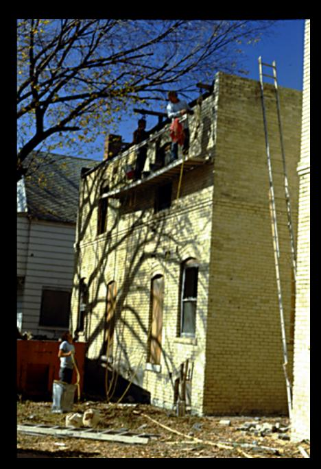
Replacement of those rotten ceiling joists has begun.
