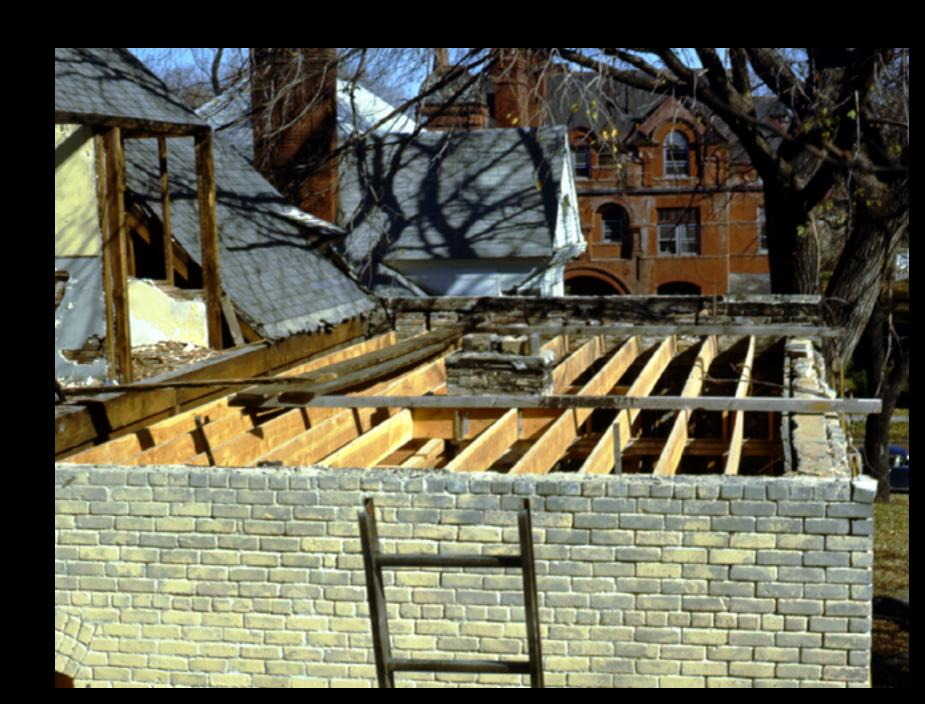
A complete gutting of the interior was followed by extensive reframing. Here, the atrium framing has been completed.
